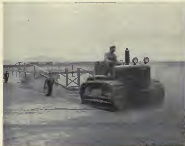
LAND LEVELING by "Landplane" on J. F. D'Ewart's unit, Pasco area, Columbia Basin project.
